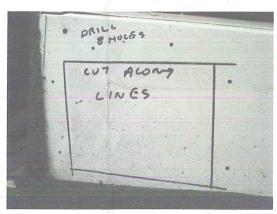
PIC. 3 Measure in 15mm from holes and draw a square to suit body of safe. Panel is aluminium and can be cut by any common means (angle grinder, jig saw with course blade, tin snips etc.). Check fit of safe, clean any sharp rough edges, place into position.
